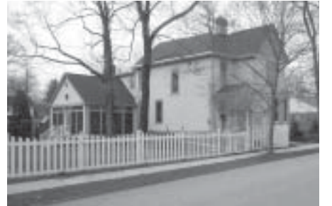
615 Amherst Avenue as it was before Hurricane Ike.
