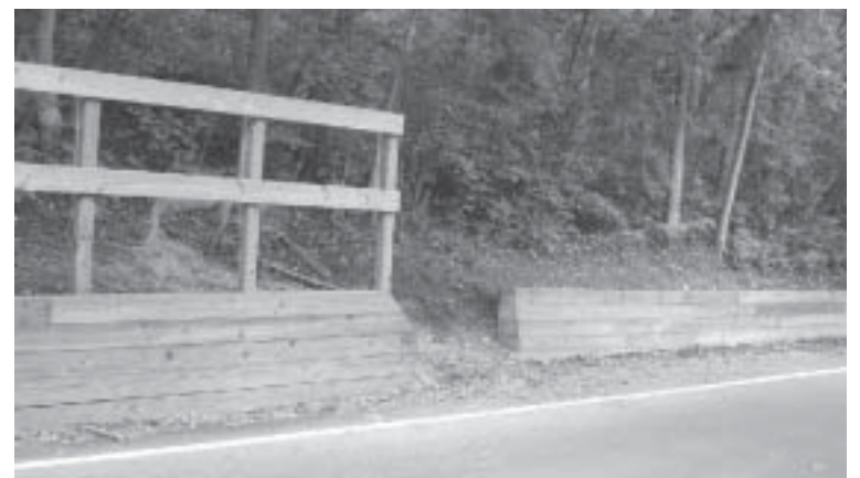
Completed Retaining Wall on Elm Avenue near the Tunnel
